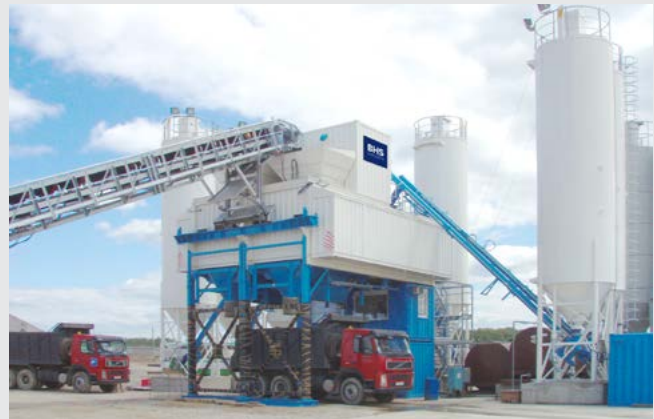
TWINMIX 3.00 in use at an airport construction project
