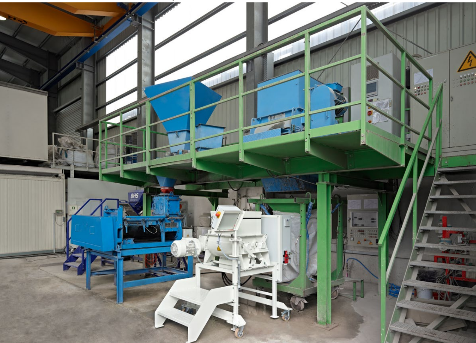
BHS technical center in Sonthofen for customer-specific testing
